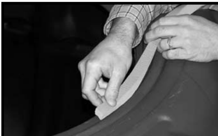
FIG.2 Apply Gasket
